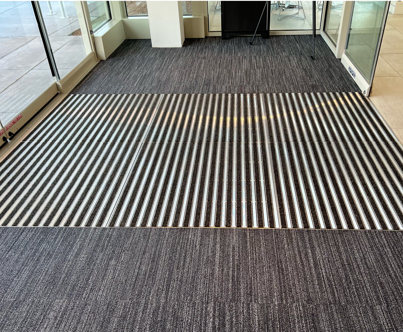
Deep recessed system with aluminum scraper bars and matting inserts
